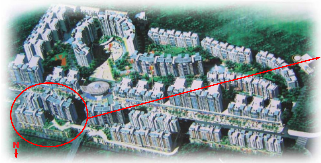
Left: Another view of Project Five. Phase One of this project is circled in red.
