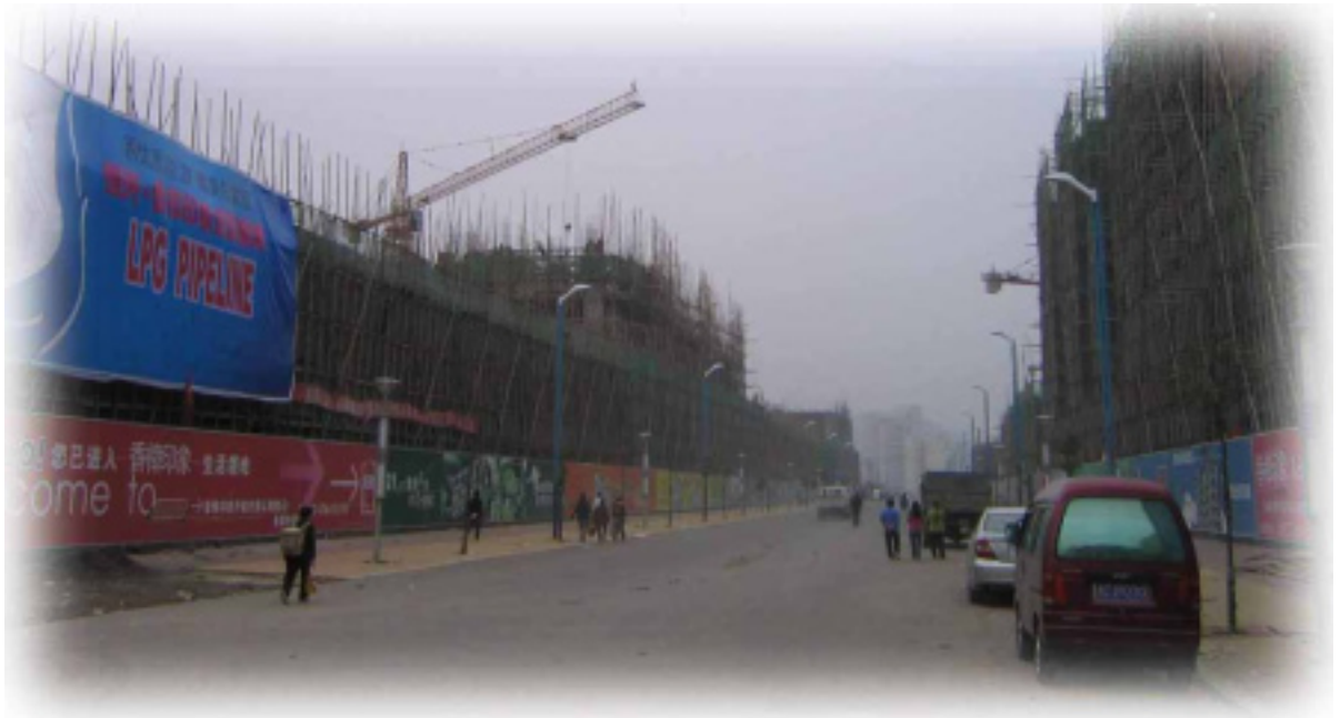
Right: Actual photo of Phase One of Project Five in progress.
